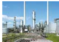
Material Testing & Inspection
