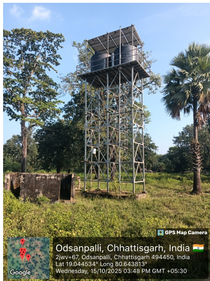
Solar-powered elevated water storage tower with two tanks in Odsanpalli, Chhattisgarh, supporting reliable rural drinking water supply.
