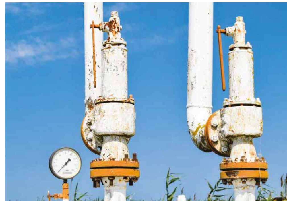
Relief valve with pressure gauge
