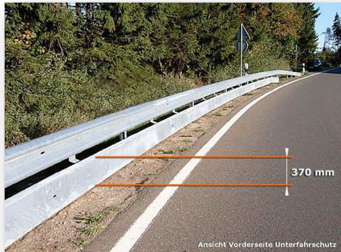
Guard Rail for motorcycle driver
