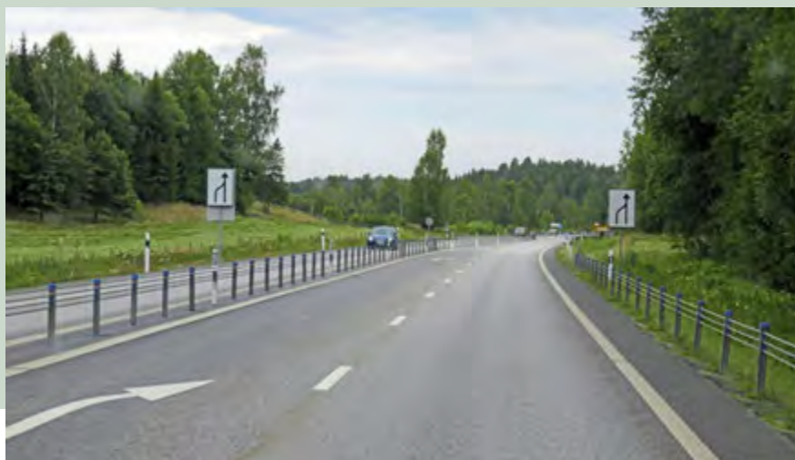
2+1 roads have proven effective in numerous countries worldwide. However, motorcyclists may be at high risk of injury if they crash into the barriers between the carriageways in each direction.
