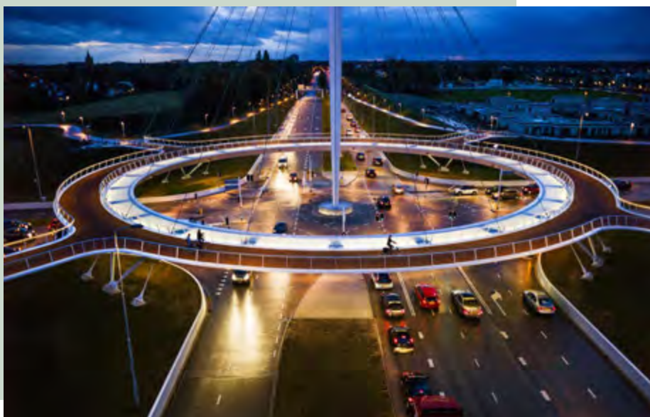
Suspended from a 70-meter pylon using 24 cables, the “Hovenring” cycle path traffic circle located between the Dutch cities of Eindhoven and Veldhoven provides around 5,000 cyclists a day with a safe means of crossing a busy intersection.
