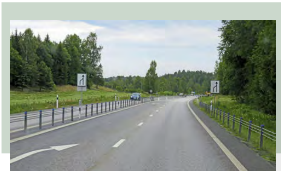
2+1 roads have proven effective in numerous countries worldwide. However, motorcyclists may be at high risk of injury if they crash into the barriers between the carriageways in each direction.
