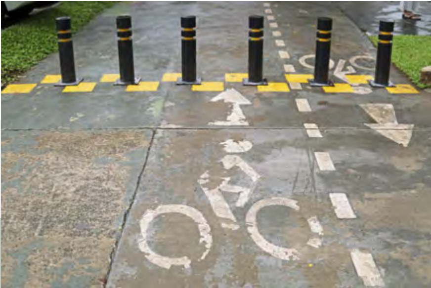
Bollards in the middle of bicycle paths are not a good solution.
