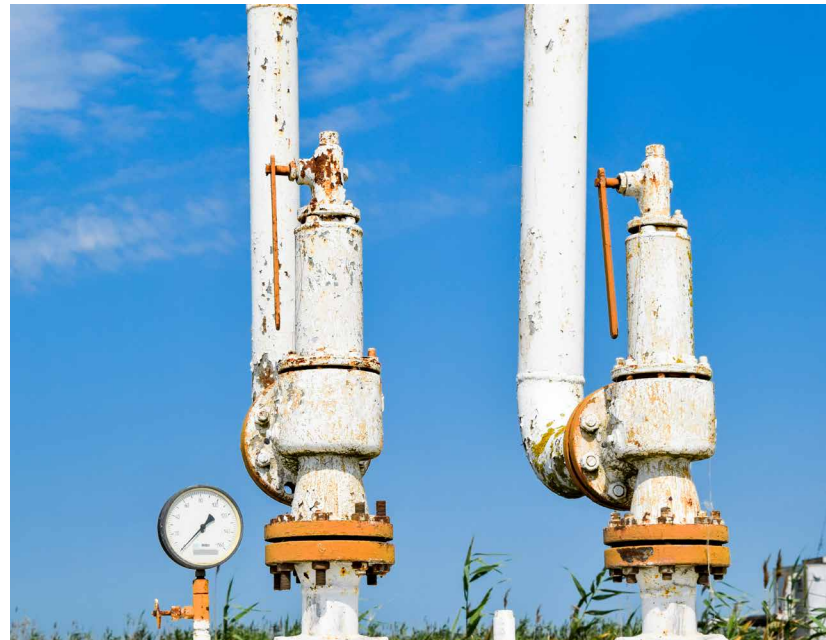
Relief valve with pressure gauge
