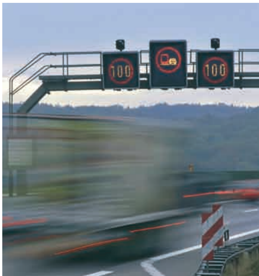
Traffic management systems can help lower the risk of accidents.
