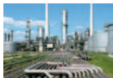
Energy and Process Industries
