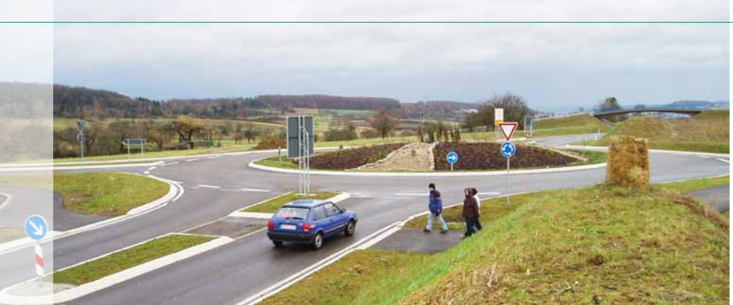
Road safety must not be neglected when creating roundabouts.
