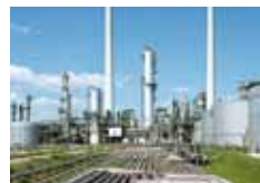
Material Testing & Inspection
