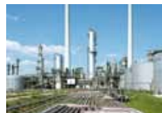
Material Testing & Inspection
