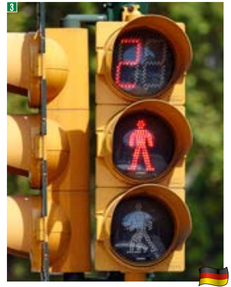
Pedestrian light with additional display showing the amount of time left before the light turns green
