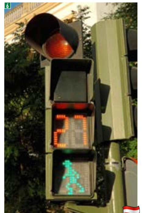
Pedestrian light with amber light informing pedestrians how much time they have left to cross the road
