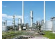
Material Testing & Inspection
